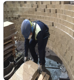
Exoskeleton 1: Picture of the first type of exoskeleton that was developed, for an operator that is mounting bricks in a squatting position.
