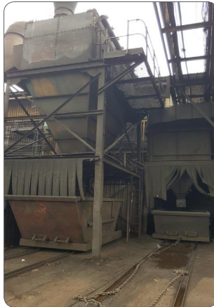
Figure 3: Shot blaster dust collection
